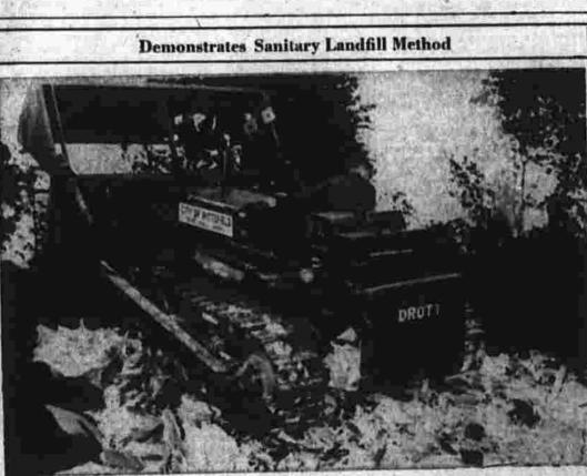
landfill method of garbage and rubbish disposal, pushes his 'dozer up a mound he has already ubbish in the compacting stage of the method. After the rubbish and garbage is fa- and over a load spread and compacted, it is covered with a two-foot layer of dirt. The domonstration, held in yesterday's downpour at the town dump, was staged for officials from all parts of the state who that morning during the past two years fro had attended a conference on the method in the Verplanck School auditorium,
